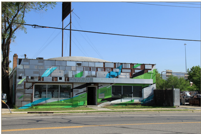
A grant secured by the Economic Development Division gave two University of Utah architectural students, Jeffrey Baird and Robert Tranter, the opportunity to realize their façade improvement project for Andrus Sales & Services at 708 West 900 South. The materials used in the renovation were recycled from Andrus' inventory.
